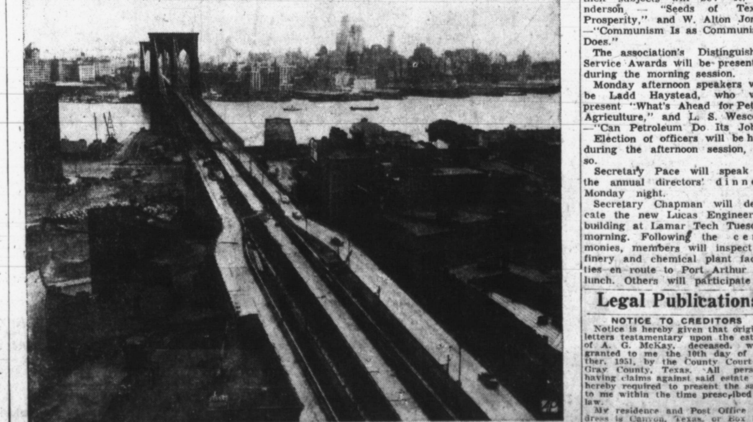
KEEPING AN OLD LANDMARK GOING — View of famed Brooklyn Bridge from lower Manhattan, N. Y., shows extensive repair work being done on approaches and structure.
