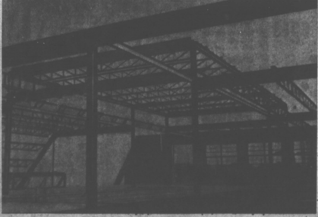
STEEL FRAMEWORK — Above is shown the steel framework for The Pampa Daily News' building. The highest, upper "center" of the building, is the ceiling for the composing room. Skylights were put along the sides. (News Photo)
