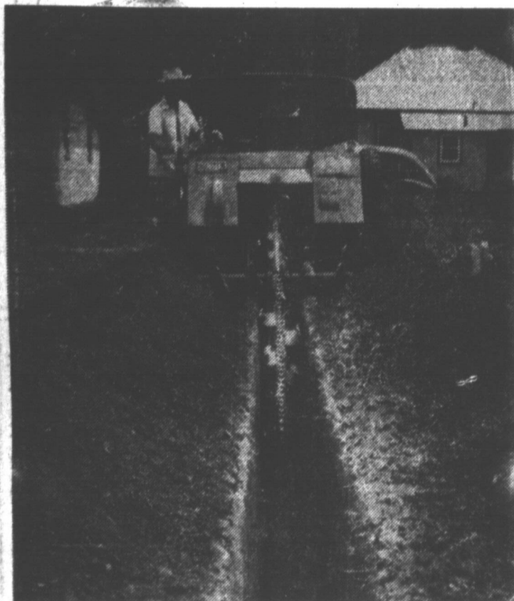
BREAKING GROUND — This was the initial phase of construction as The Pampa Daily News began its new plant. Holes for concrete pillars later were drilled in this trench, foundation forms erected and the foundation poured. This picture was taken as the trench was being cut for the south end of the building. (News Photo)
