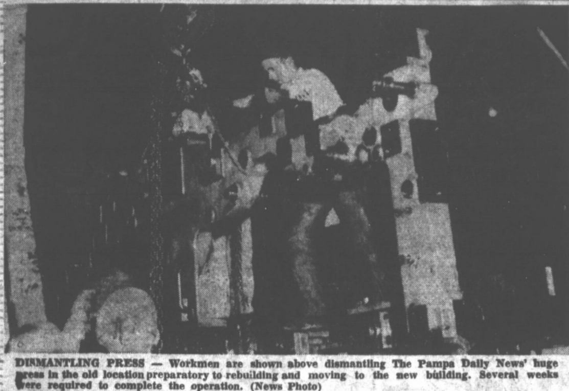
DISMANTLING PRESS — Workmen are shown above dismantling The Pampa Daily News' huge press in the old location preparatory to rebuilding and moving to the new building. Several weeks were required to complete the operation. (News Photo)
