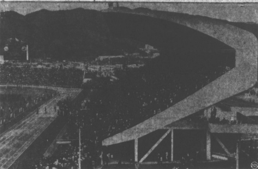
DEDICATION—This was the general view of the brand new Olympic Stadium, Caracas, as the athletes of Venezuela, Bolivia, Colombia, Ecuador and Panama, competing in the Bolivarian Games, paraded. It accommodates 35,000. The stand is of the cantilever style, no posts. The Games run through Dec. 21. (NEA)
