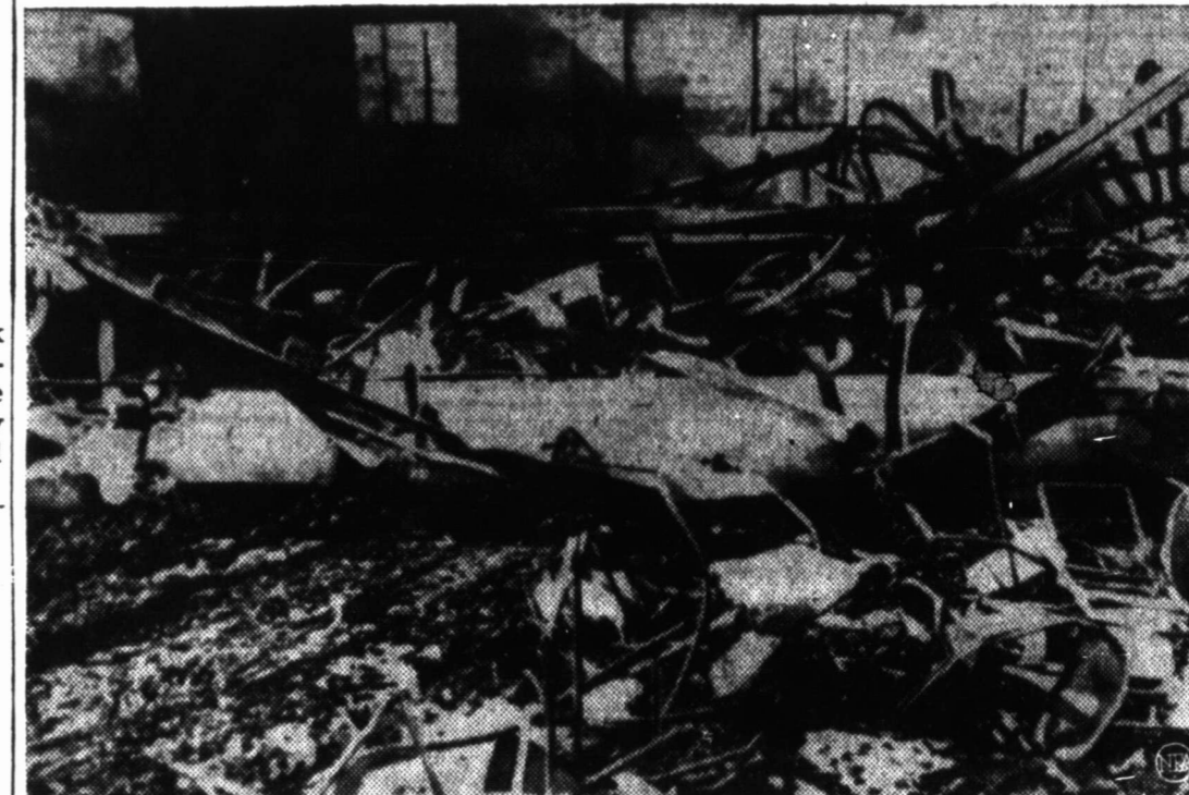
CHRISTMAS PARTY HOLOCAUST — Twisted steel girders and broken chairs are all that remains of the Civic Auditorium, Tijuana, Mexico which went up in flames taking at least 41 lives. A short circuit in wire lighting Christmas decorations caused the blaze. (NEA TELEPHOTO)
