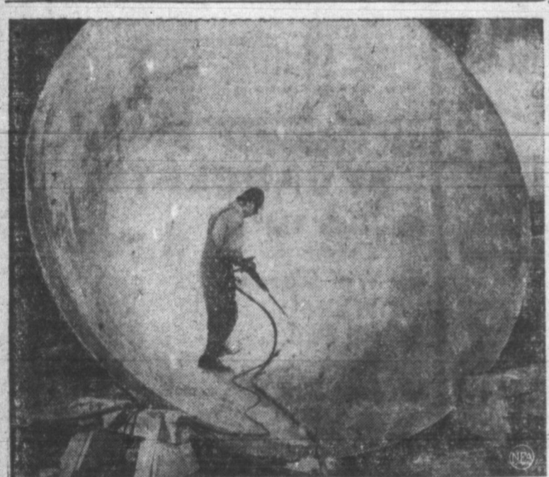
WELL POTTED—Paul S. Gable hammers away at finishing touches on world's largest cast steel cinder pot, fabricated by U. S. Steel, for new works at Morrisville, N. J. The 10 1/2-foot deep pot, 12 1/2 feet across the mouth, will handle 42,600 pounds of hot slag.
