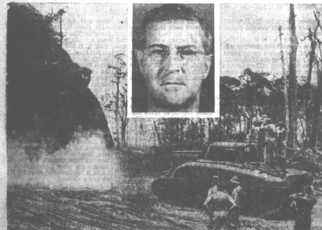
Exasperated by the tedious hours it took for a six-man crew to drill holes for blasting a roadway through a volcanic hill at a Pacific base, Chief Carpenter's Mate Thomas J. Waters (inset) of Arlington, Mass., got the bright idea of pumping 75-mm. shells from a Marine Corps General Sherman tank into the hill.
