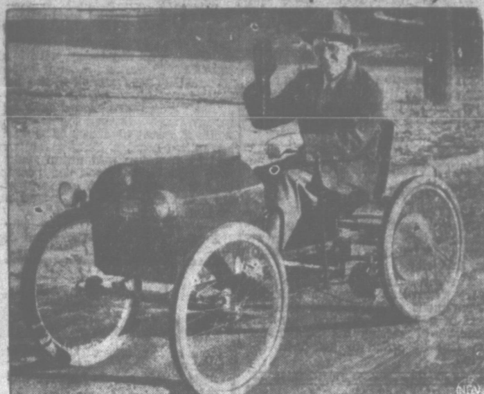
Gas rationing doesn't bother Joseph Jacobs, above, Minneapolis electric company superintendent. He drives to work in this electric car he built during his spare time. With four speeds forward and four reverse, it operates on three 12-volt storage batteries and makes 15 miles an hour and 100 miles to the battery charging.
