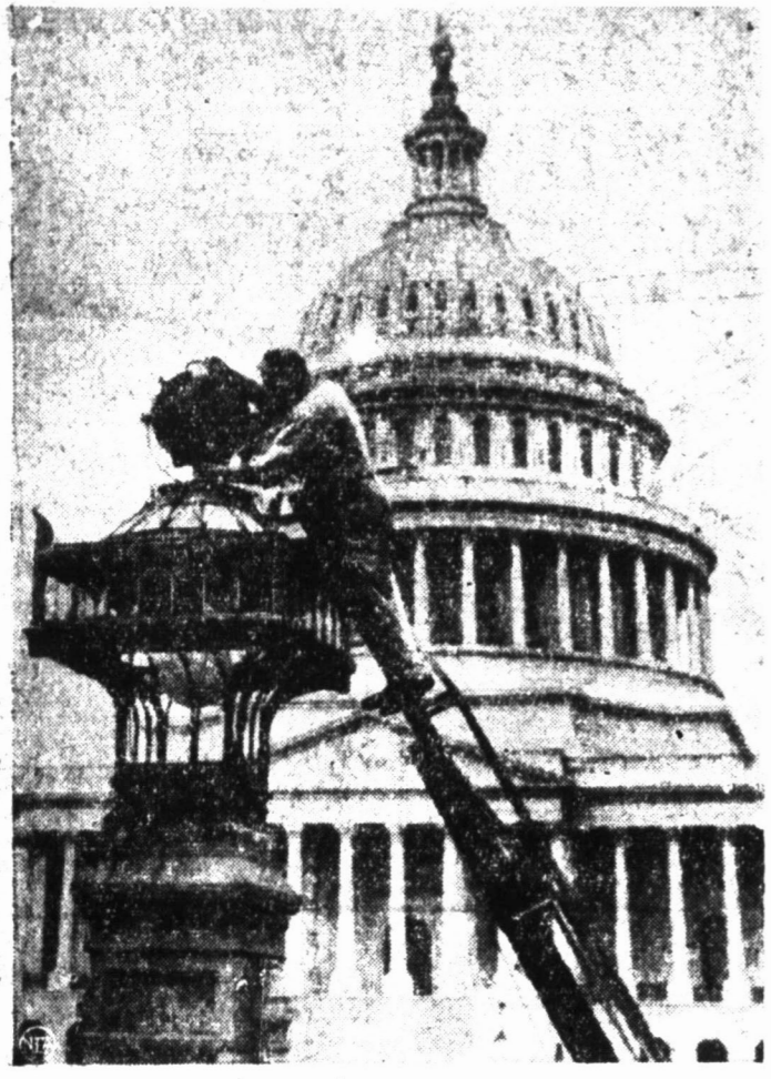
Washington is getting all dolled up to celebrate the coming victory over Germany. Capitol dome, in background of photo above, has just been repainted. Workmen in foreground is fixing up a floodlight that will illuminate the dome when news comes that V-day is here.
