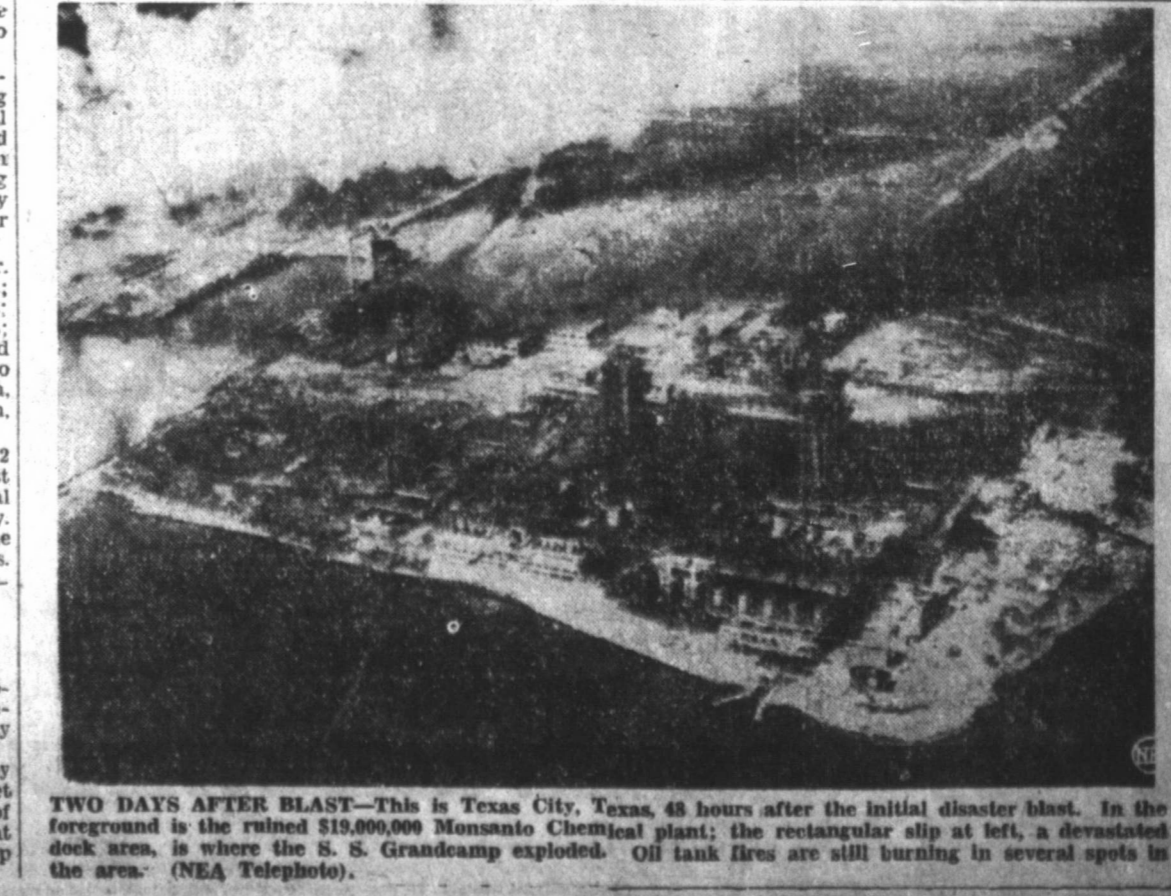
TWO DAYS AFTER BLAST—This is Texas City, Texas, 48 hours after the initial disaster blast. In the foreground is the ruined $19,000,000 Monsanto Chemical plant; the rectangular slip at left, a devastated dock area, is where the S. S. Grandcamp exploded. Oil tank fires are still burning in several spots in the area. (NEA Telephone)
