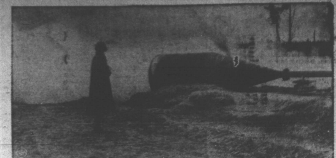
MUFFLER FOR NATURE'S STEAM —Wairakei, in northern New Zealand, has long been a resort and is also rich in underground steam pockets which scientists are now exploring in an attempt to harness the steam for electric power. But the roar of the escaping steam is so great that it would keep hotel guests awake, so a giant muffler has been placed on each test bore to lessen the noise. The volume of sound is reduced by allowing the steam to expand before escaping.
