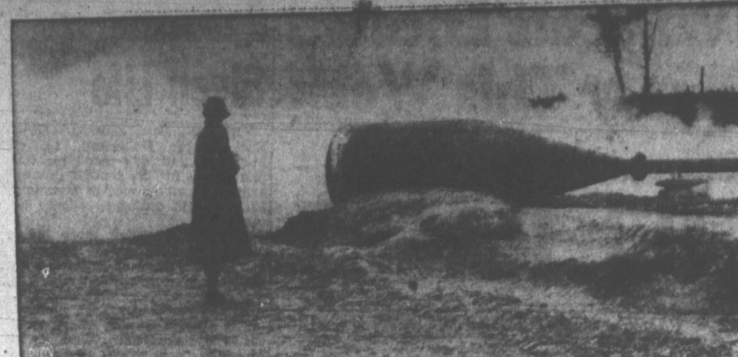
MUFFER FOR NATURE'S STEAM—Wairakei, in northern New Zealand, has long been a resort and is also rich in underground steam pockets which scientists are now exploring in an attempt to harness the steam for electric power. But the roar of the escaping steam is so great that it would keep hotel guests awake, so a giant muffer has been placed on each test bore to lessen the noise. The volume of sound is reduced by allowing the steam to expand before escaping.
