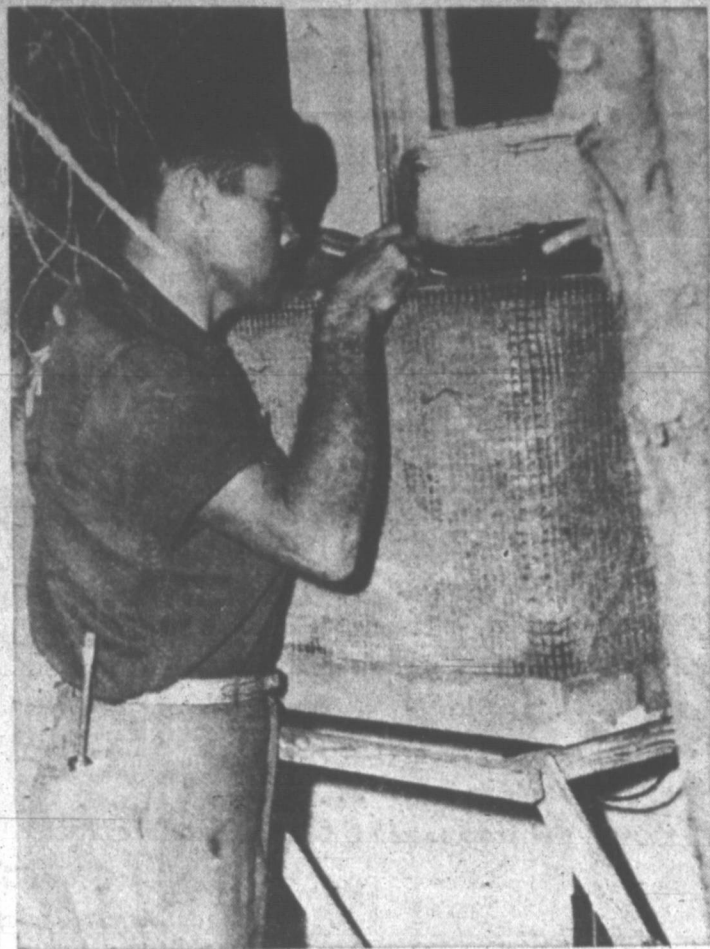
IT'S WARM WORK, installing an air conditioner. Robert Fewell, a service man at Bert A. Howell Inc., has been installing coolers for several years, but he believes this year the conditioners are giving better service than ever due to the extremely dry atmosphere. (News Photo)
