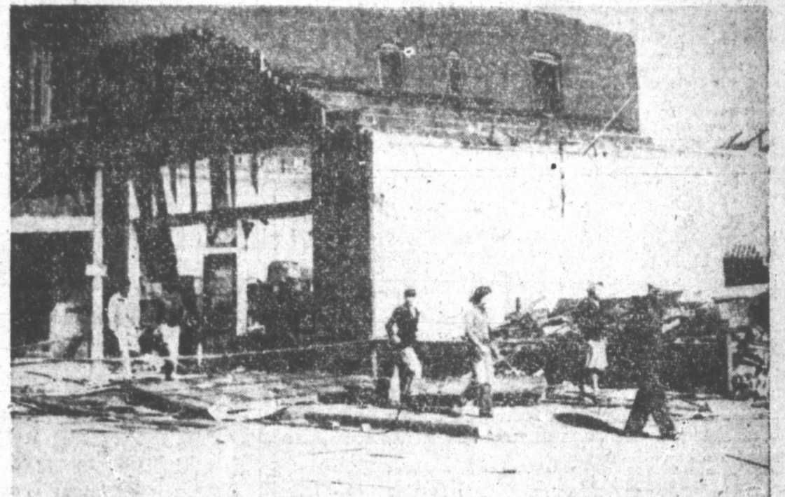
DAMAGE GREAT IN TORNADO —Stores and homes alike were destroyed or damaged in Woodward, Okla., when a tornado struck the town. No estimate has been advanced on amount of property loss suffered.
