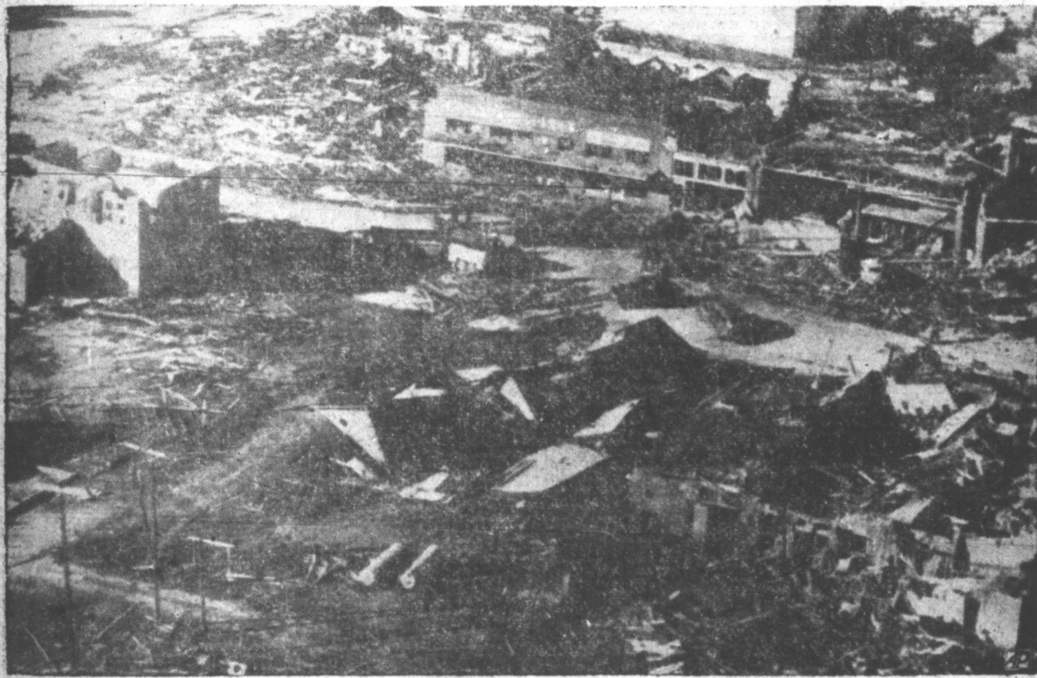
BUSINESS DISTRICT AFTER STORM —This is a portion of the wrecked business district of Higgins, one of the several towns struck by a tornado which left death and destruction. This picture was made from the air.
