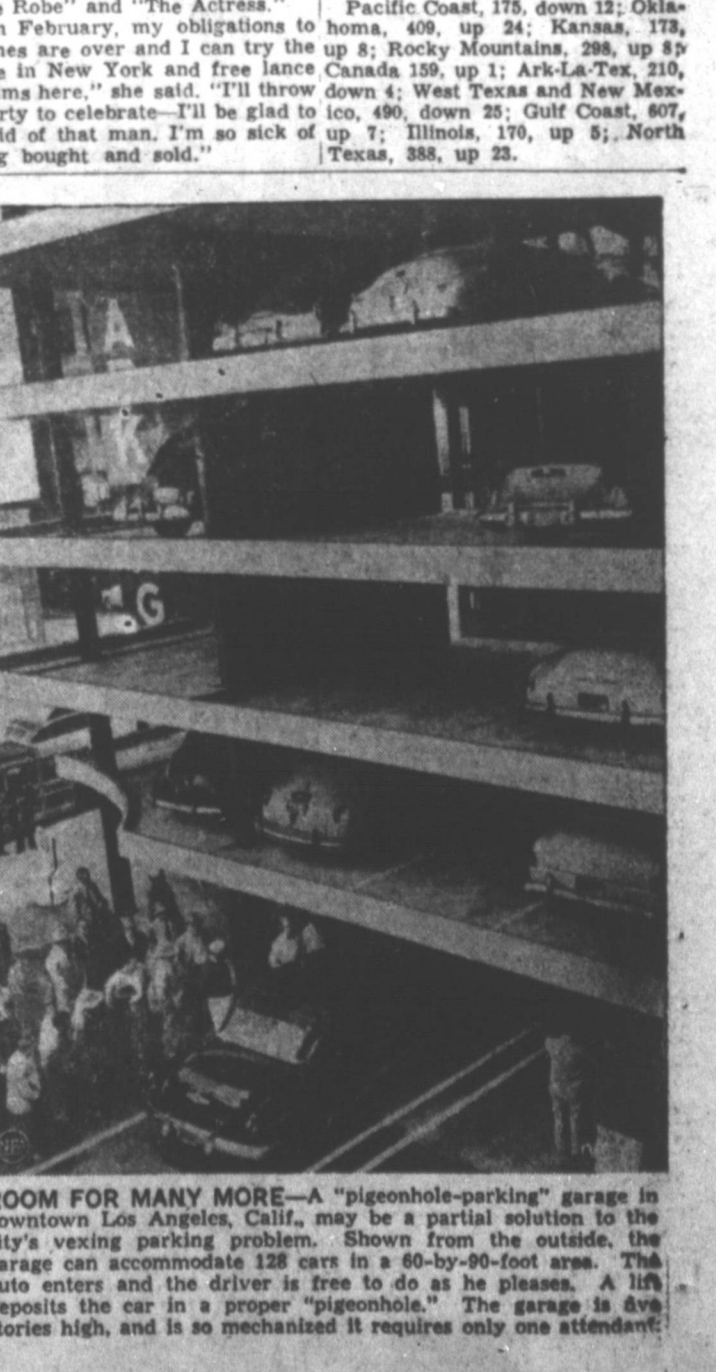
ROOM FOR MANY MORE - A "pigeonhole-parking" garage in downtown Los Angeles, Calif., may be a partial solution to the city's vexing parking problem. Shown from the outside, the garage can accommodate 128 cars in a 60-by-90-foot area. The auto enters and the driver is free to do as he pleases. A lift deposits the car in a proper "pigeonhole." The garage is five stories high, and is so mechanized it requires only one attendant.
