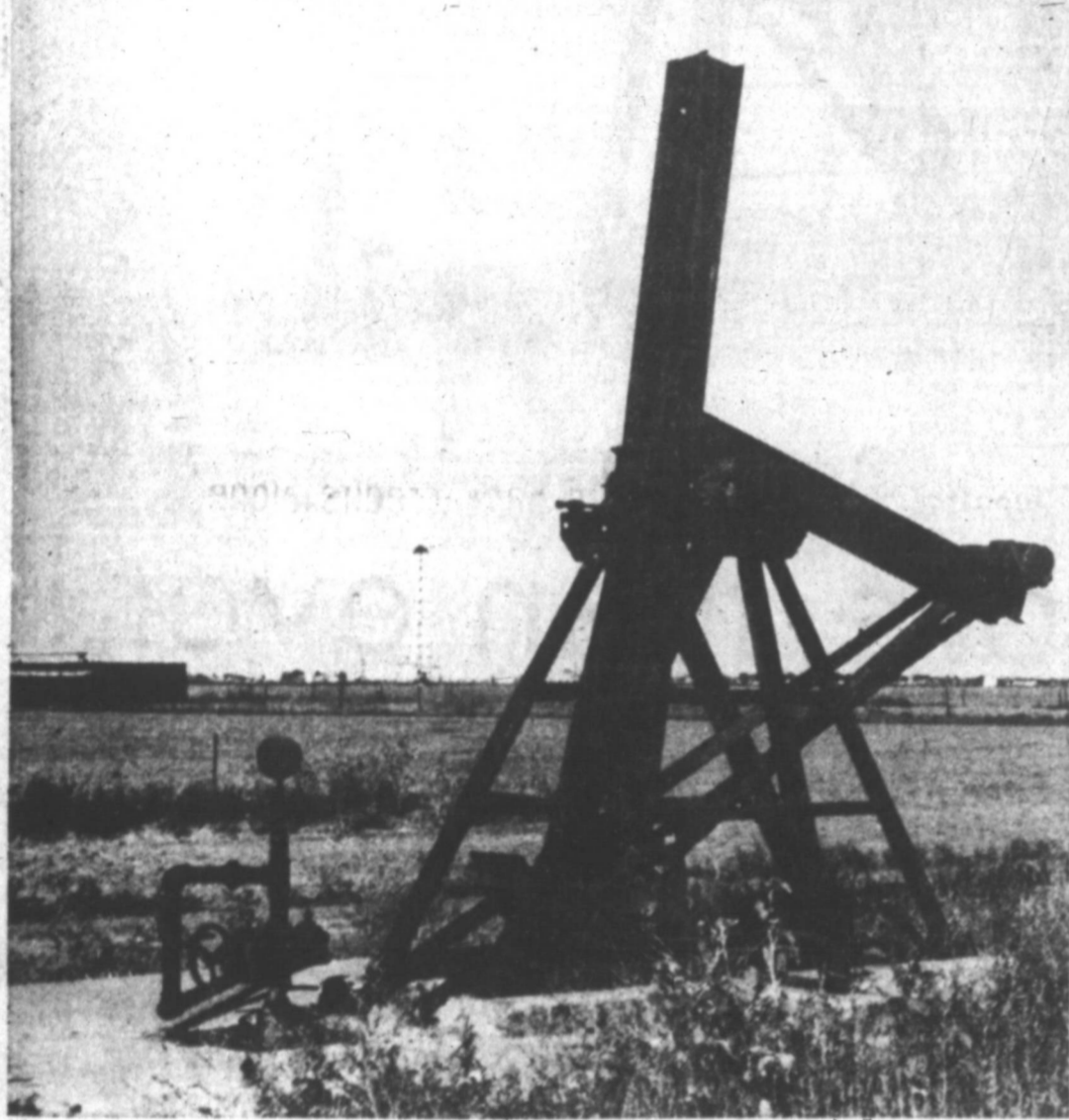
INJECTION WELL — One of the 162 gas injection wells in the West Pampa oil field is pictured above at the left of the pump jack of the Southern Petroleum company well No. 14 on the Vaughn lease. This injection well, one of the first to be drilled here, was placed in service on the first day of gas injection in the field on March 25, 1946. The well is used to inject gas into the oil well so that more than the normal amount of oil might be pumped from the hole.
