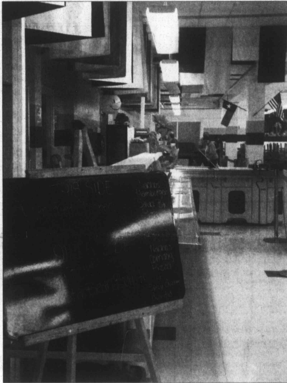
The current Pampa High School cafeteria, built in 1941, will be torn out this summer and classrooms will be installed in the space. A new cafeteria will be built upstairs by the new commons entrance of the high school.
