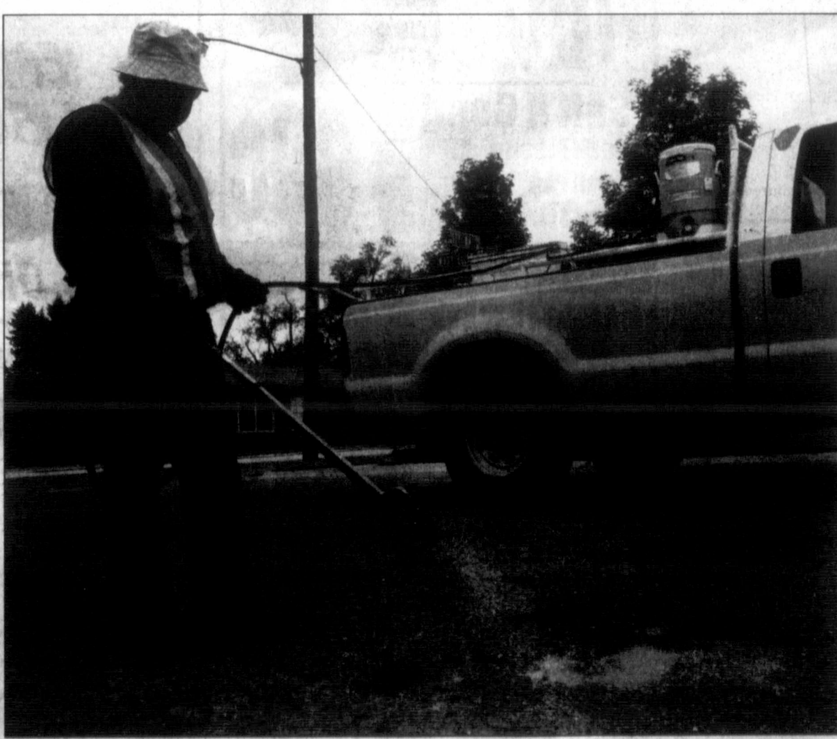
staff photo by David Bowser Lighting up the streets of Pampa, Benito Reynaga with Lewis Construction uses a propane torch to heat the asphalt in the 1700 block of Mary Ellen in preparation for the city's annual seal coating project.
