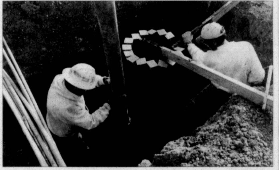
Gregg Story (left) and Hank Nunn with Brundage Bone Concrete Pumping pour the concrete footings for base of the bowl slide at Pampa's water park. The park is expected to be open by next summer.
