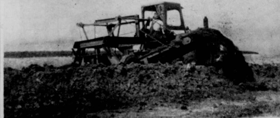
TERRACE EXPERT—Nat Bradley is shown above building a terrace on the Bill Kilpatrick farm, about three miles southeast of Memphis. Bradley, who works in Hall and Donley Counties, expects to build 50 or more miles of new terraces before September 15. The Hall County Soil Conservation crew runs the lines for the terraces and government assistance is given the farmers through the AAA office here. (Photo Courtesy Amarillo Times)
