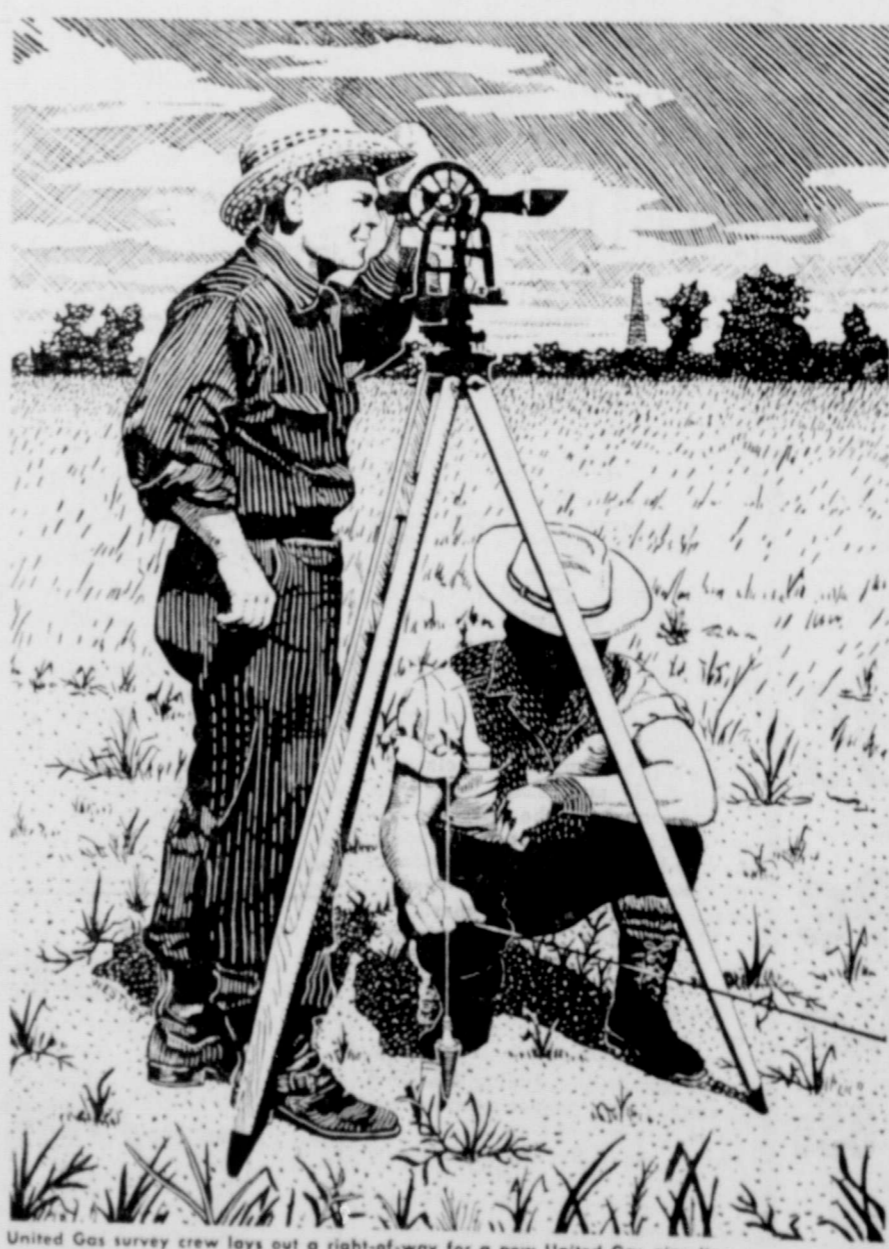
United Gas survey crew lays out a right-of-way for a new United Gas pipe line
