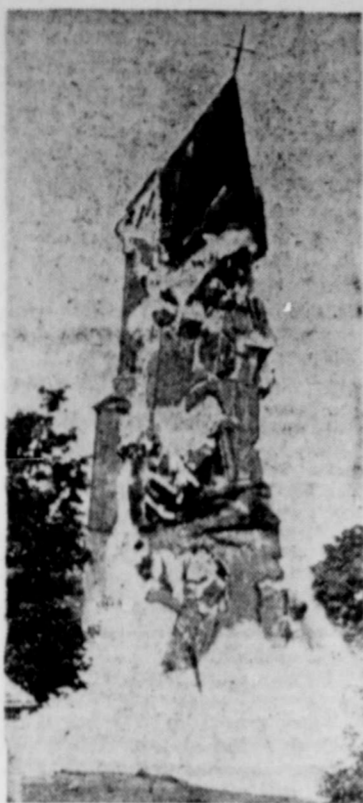
STEEPLE TOPPLES . . . Steeple of St. Sebastian, Ludwigshafen, Germany, is dynamited after being declared unsafe.
