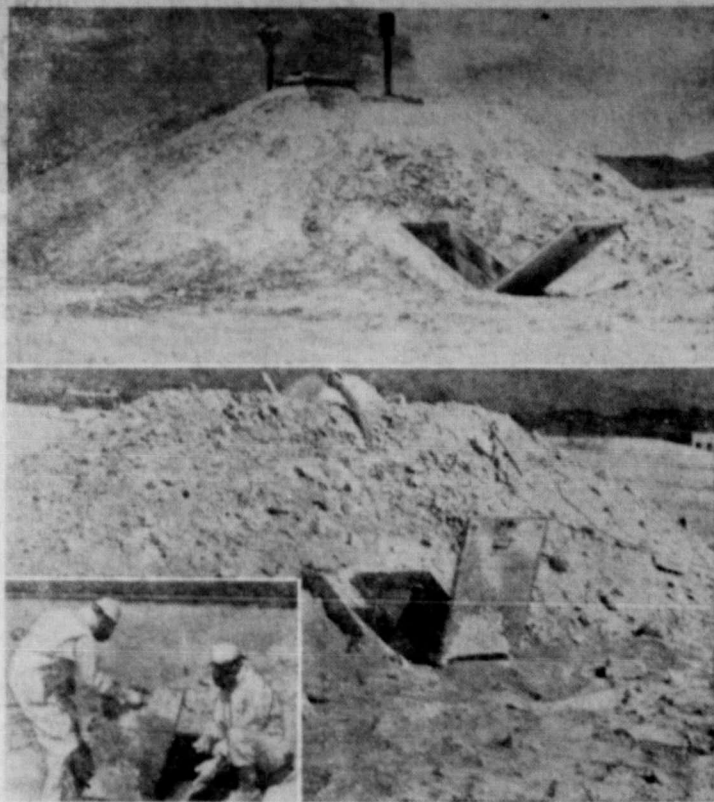
HOME SHELTER of reinforced concrete (top) at the Operation Plumbbob atomic tests in Nevada withstood a blast pressure of some 65 pounds per square inch (bottom) with damage only to vent pipes (the average house can withstand a pressure of about one pound per square inch). The shelter, which could accommodate about six persons, was covered with 5 1/3 feet of earth for near-complete protection against initial radiation in blast areas. When specially-dressed radiological monitors (inset) entered the area after the A-blast, they found the steel plate door undamaged and easily opened with normal pressure.
