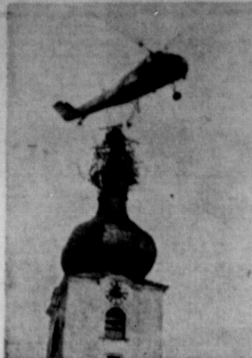
GOOD DEED . . . U. S. army helicopter hoists 200 pound cross to top of church steeple in Konnersreuth, Germany.
