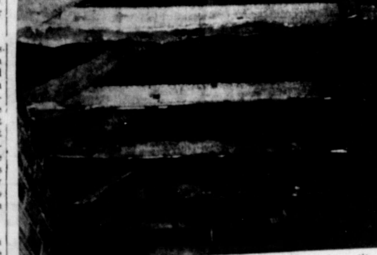
CEILING DAMAGE — Pictured above is part of the ceiling of the Memphis Frozen Food Locker which was damaged by fire Sunday afternoon. Firemen spent an hour battling the blaze.
