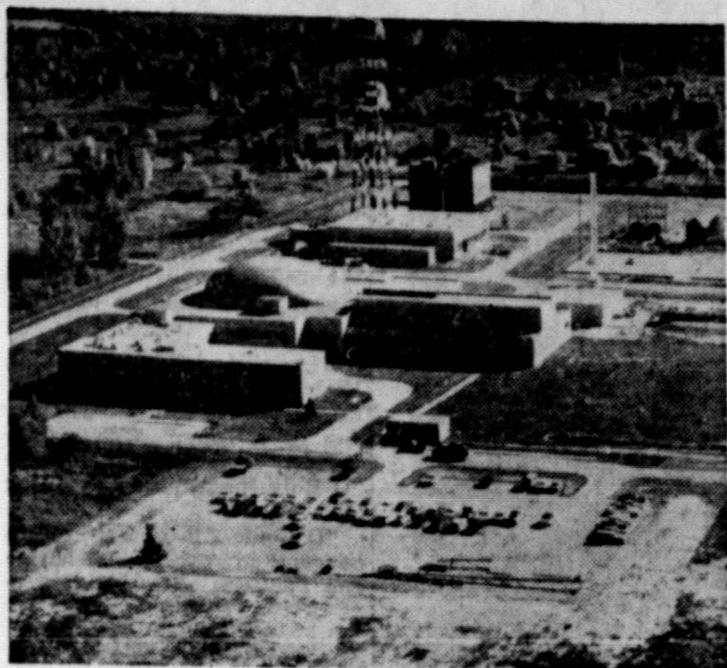
HOUSE OF SCIENCE... Newly-completed Plum Brook Reactor Laboratory, nuclear reactor station, rises in rural area of Northern Ohio. Dome structure contains nuclear reactor.
