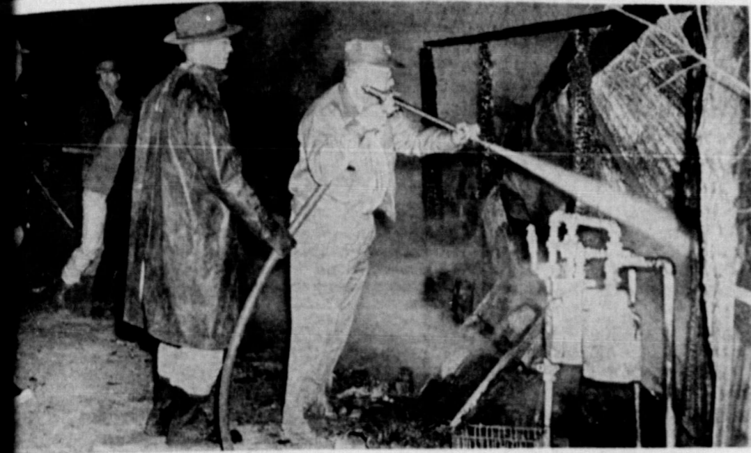
DESTROYED — Firemen Monday night fought a fire in a home at Morningside but structure was almost completely destroyed before it could be brought under control. Seen in this picture include H. E. Craig, left, Will Leslie, center, and O. R. Saye. In background is Charlie Grice; and Pat Johnson and Jimmy Winters with the pole moving the burned material aside.
