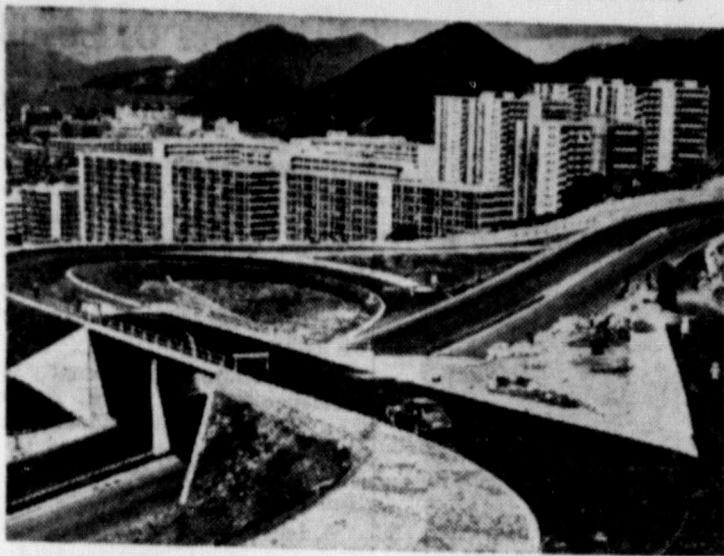
OLD FOOTHILLS ROAD . . . Highway traffic problems are eased in Hong Kong with the opening of this new clover-leaf section on the New Lung Cheung Road, formerly the Kowloon Foothills Road.
