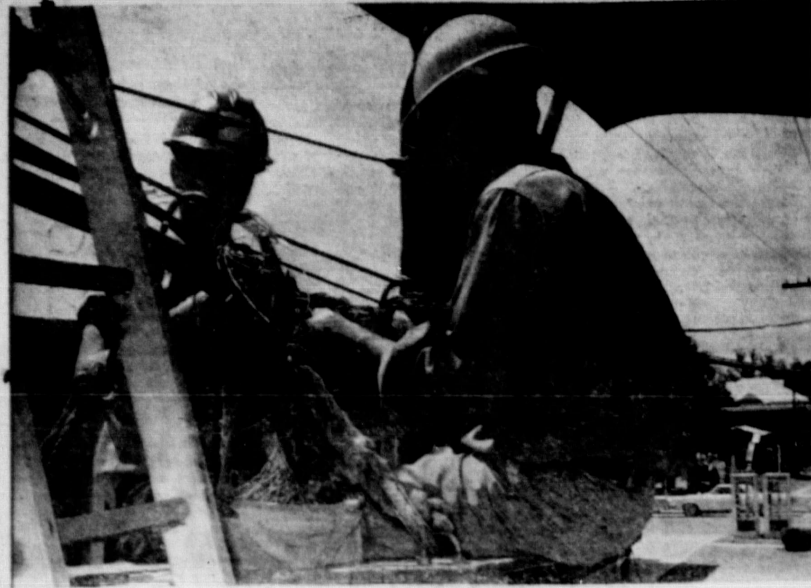
CABLE SPLICING—Larry Crump (left) and Donald James (right), cable splicers for General Telephone Company of the Southwest, work high above the street putting the finishing touches on a major telephone cable addition in Memphis.
