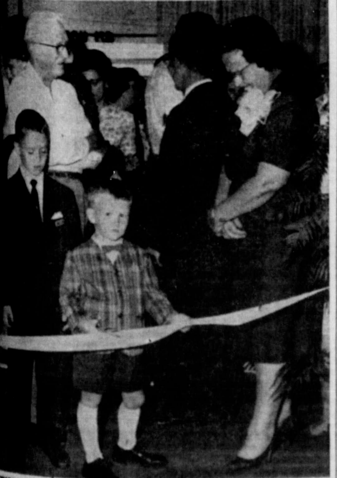
CUTTING RIBBON —Shown above is Chip Martin, 5-year-old son of Mr. and Mrs. Malcom Martin, as he prepares to cut the ribbon opening the new First State Bank building for public display. Beside Chip, is his friend, Dan Bennett, son of Dean Bennett, the construction superintendent. To the right is shown, Chip's grandmother, Mrs. L. C. Martin, wife of the bank's Executive Vice-President, L. C. Martin. The opening house Saturday afternoon was well attended by many area bankers as well as interested citizens of the entire area.
