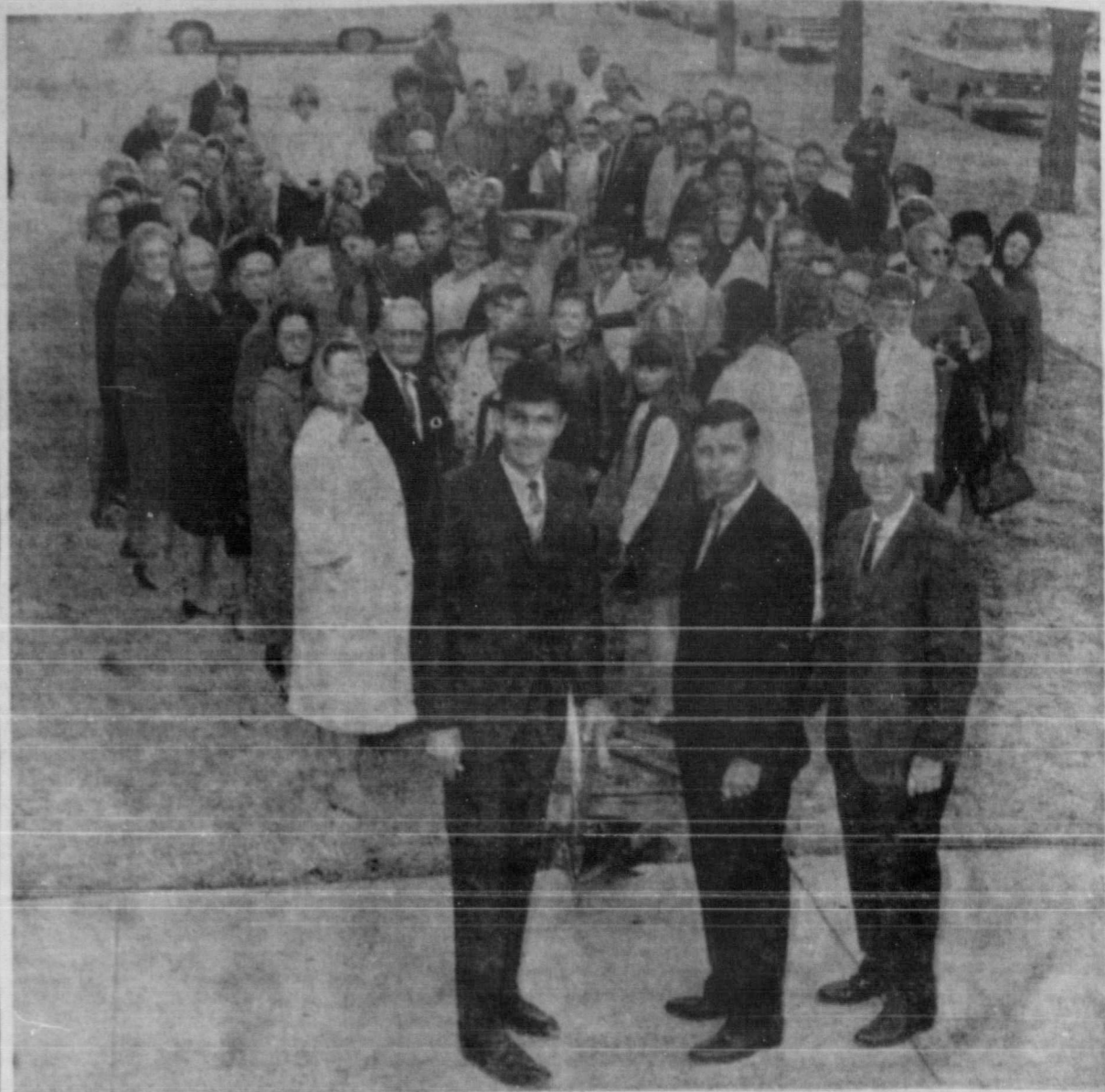
GROUND BREAKING WITH HUMAN POWER —Three groups from the membership of the First Baptist Church in Memphis participated in pulling the above pictured plow during official ground breaking ceremonies for the new home of the First Baptist Church. In the foreground are shown Rev. Gene Jorgenson, pastor of the church, who directed the ceremony, Cliff Pedersen, director of music, and J. M. Ferrel, Jr., chairman of the building committee. Youngsters, building committee members, deacons, and those members who were alive before 1900 were asked to be first to take hold of the ropes, and then others were asked to join in before the plow was pulled through the front lawn at the spot where the new nursery room of the church will be built. The ceremony was originally scheduled for last Sunday morning but adverse weather caused the postponement.
