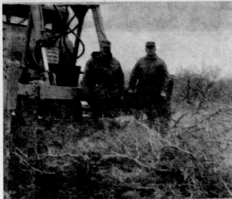
RANGE BRUSH CONTROL —Jerry Smith, contractor, and L. F. Widener, farmer, are shown above on a farm southwest of Memphis where brush control is being done by root plowing mesquite in poor condition rangeland. Land will be roller chopped and seeded to native grass.
