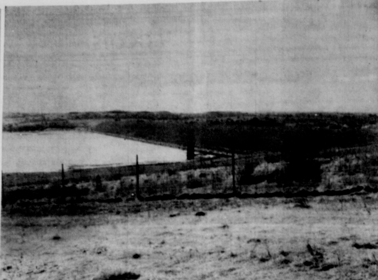
FIRST DAM COMPLETED —Pictured above is Site 4 dam, the first one completed. Shown is the fencing, riprap with rock and the lake level up to the main spillway. This dam saved the Gardenhire and other farms from flood waters this past spring when a 5-inch rain fell in Bitter Creek drainage area.
