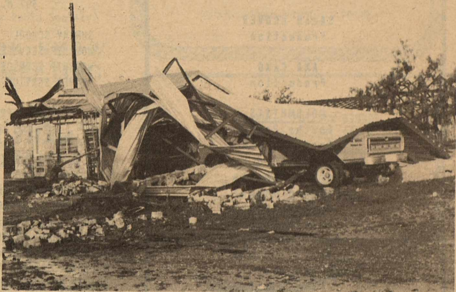
This carport at Santos & Zoila Ortiz's ranch had one vehicle pull out from under it with only one side window blown in and a few scratches. The wind picked up the rock columns holding the roof and moved them and the pickup under it a few feet away from where they were originally.
