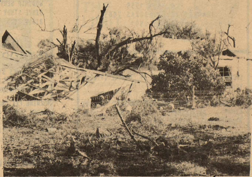
A pile of debris is all that is left of a green house that was located in the rear of the Joe York, Jr. house.
