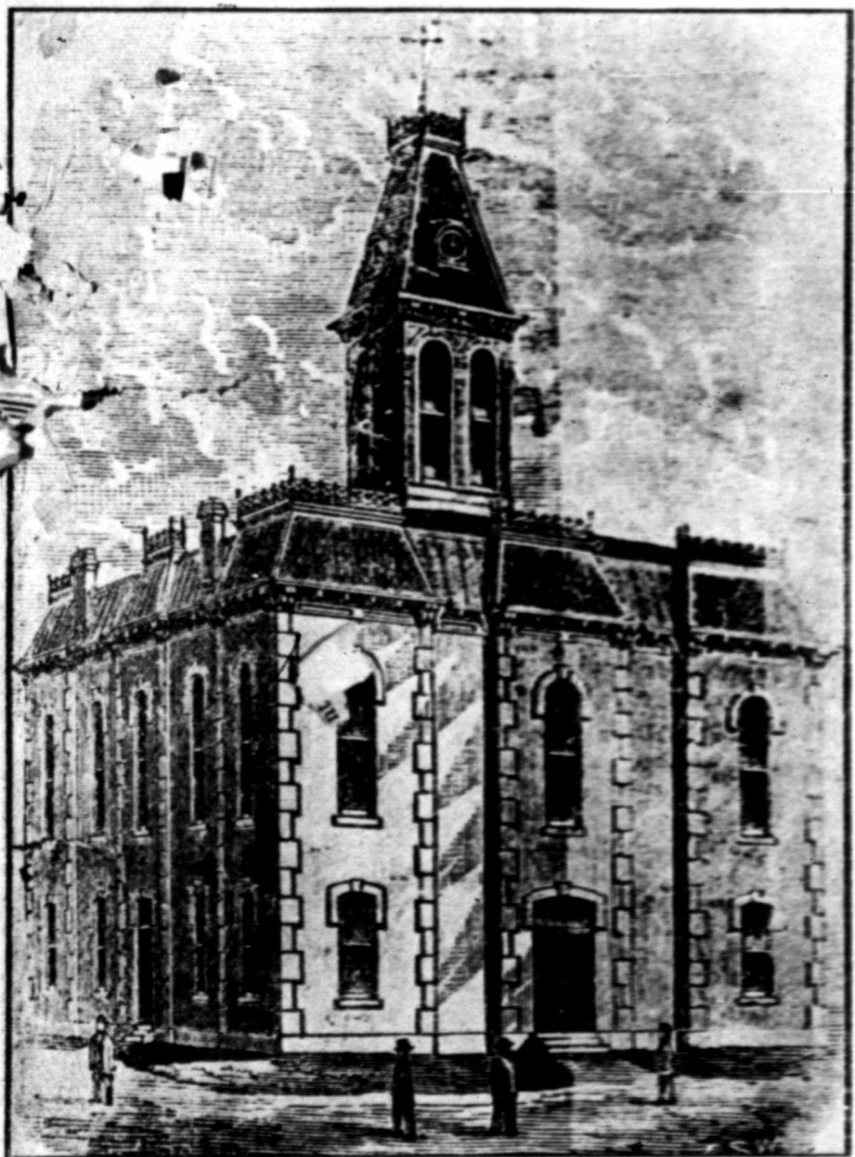
First Court House of Mitchell County which was torn down to give place to the present structure. See picture on first page.
