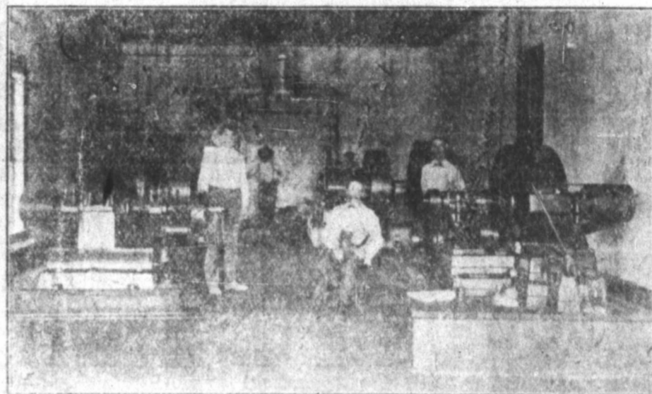
INTERIOR VIEW ELECTRIC LIGHT PLANT
