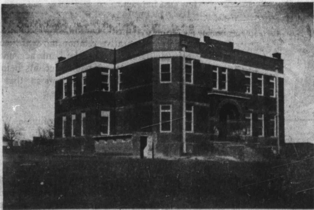
WARD SCHOOL BUILDING
