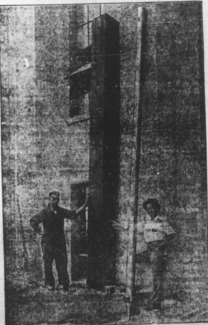
Here's the "biggest" and "littiest" pipes for the great Barton organ, now being installed in the new auditorium at the State Fair of Texas, Dallas. There are more than 3500 pipes in the big instrument, which will be heard every day during the 1925 State Fair, Oct. 10-25. The man at the right is holding the smallest pipe in his hand. It's only 3/4 inches long and about as big around as a lead pencil. The others are eighteen feet in height.
