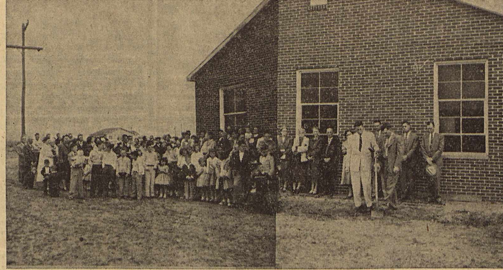
GROUND-BREAKING WAS HELD SUNDAY, March 10, for the new educational building at the First Baptist Church. The building will have 6,412 square feet of floor space, and will cost an estimated $40,000. Plans are for the building to be complete by June 15. REVIEW Photo
