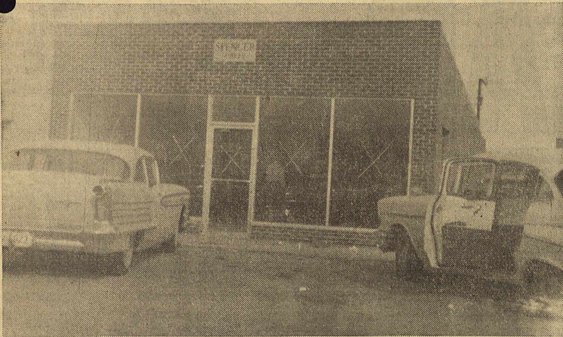
RECENTLY COMPLETED is the Spencer Building, of modern brick masonry with glass and aluminum front. The building, located next to
