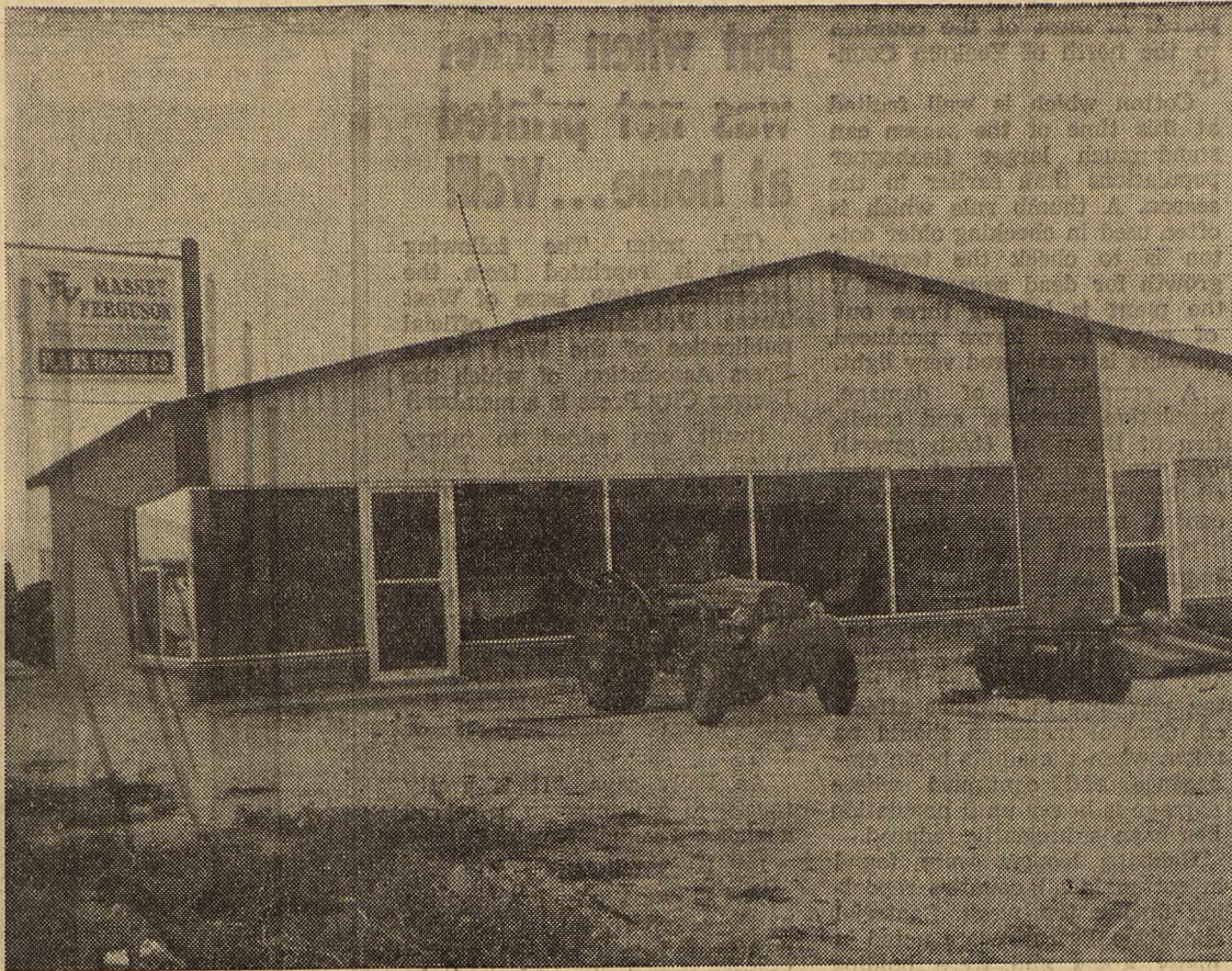
NEW BUILDING of the Plains Tractor Company was recently completed west of town. The building houses the Massey-Ferguson tractors and im-
