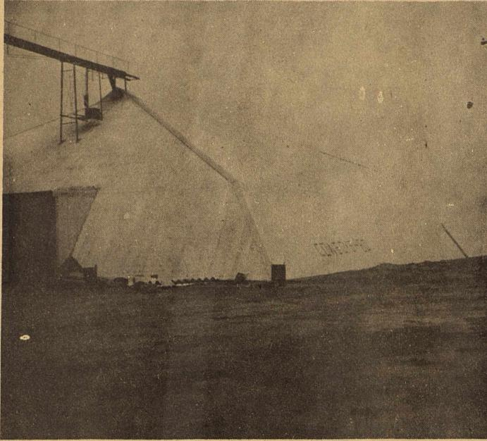
**BIG BUILDING**---One of the biggest construction jobs in the Plains area during 1960 was this huge grain storage building built by Goodpasture Grain and Milling Company. The building, with room for more than 400 million pounds of grain, is equipped with a modern dryer. Cost ran well above \$100,000.
