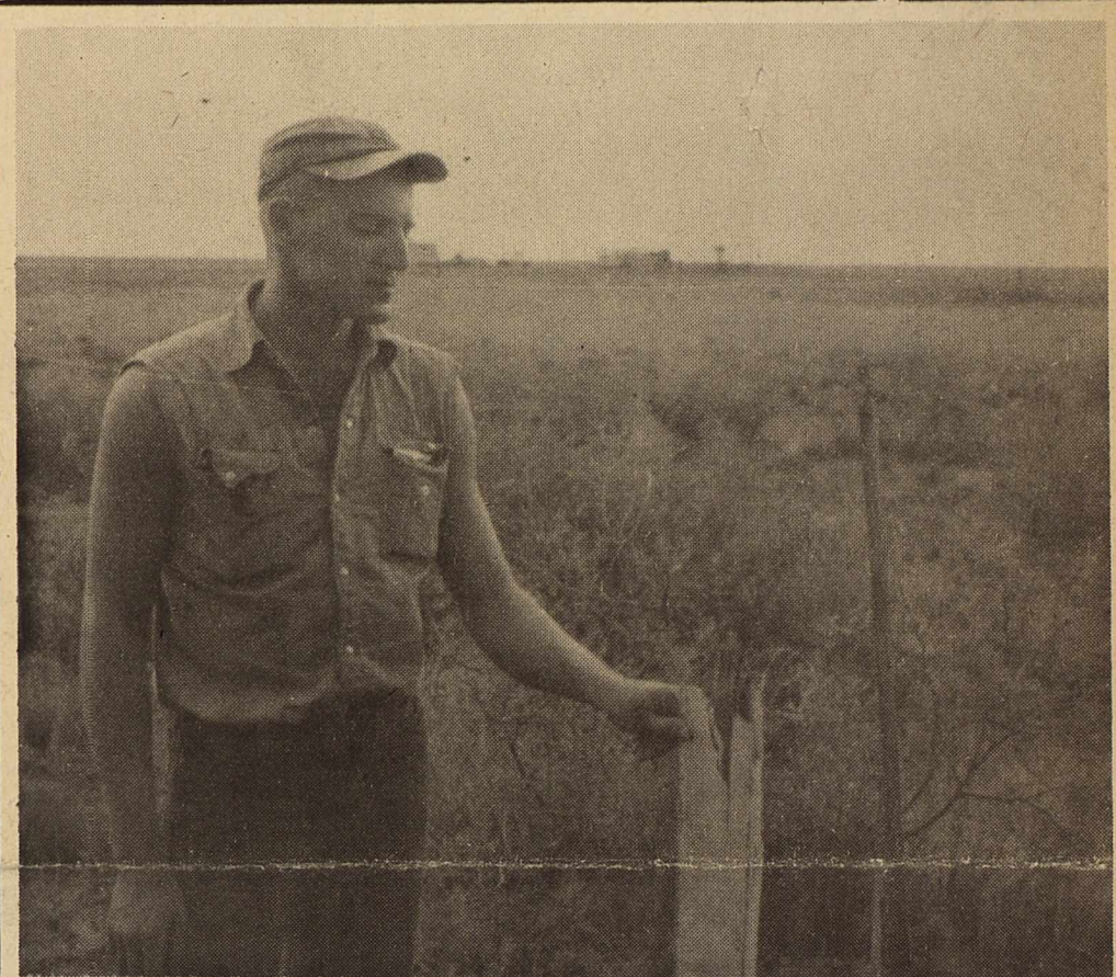
SNAPPED ---This 4x4 post supporting a highway sign was snapped in two by Wednesday's twister which passed just east of the city limits. Here, Venum Fitzgerald inspects what is left of the post. In the background is the Roy Fitzgerald home. The tornado cut its path west of the Fitzgerald home.
