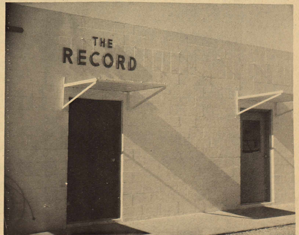
THE PLAINS RECORD---moved to new quarters in one of Plains' newer buildings, the Don Hancock bldg.
