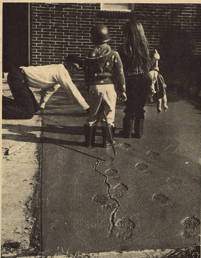
From the cement finisher's expression, it's not hard to guess what he's really thinking. But good craftsman Calvin Joiner of Brownsboro, Ala., carefully refinished this job in Southeast Huntsville after explaining to his uninvited guests that concrete becomes like rock, and their footprints would be around for 50 years or more if left there.
