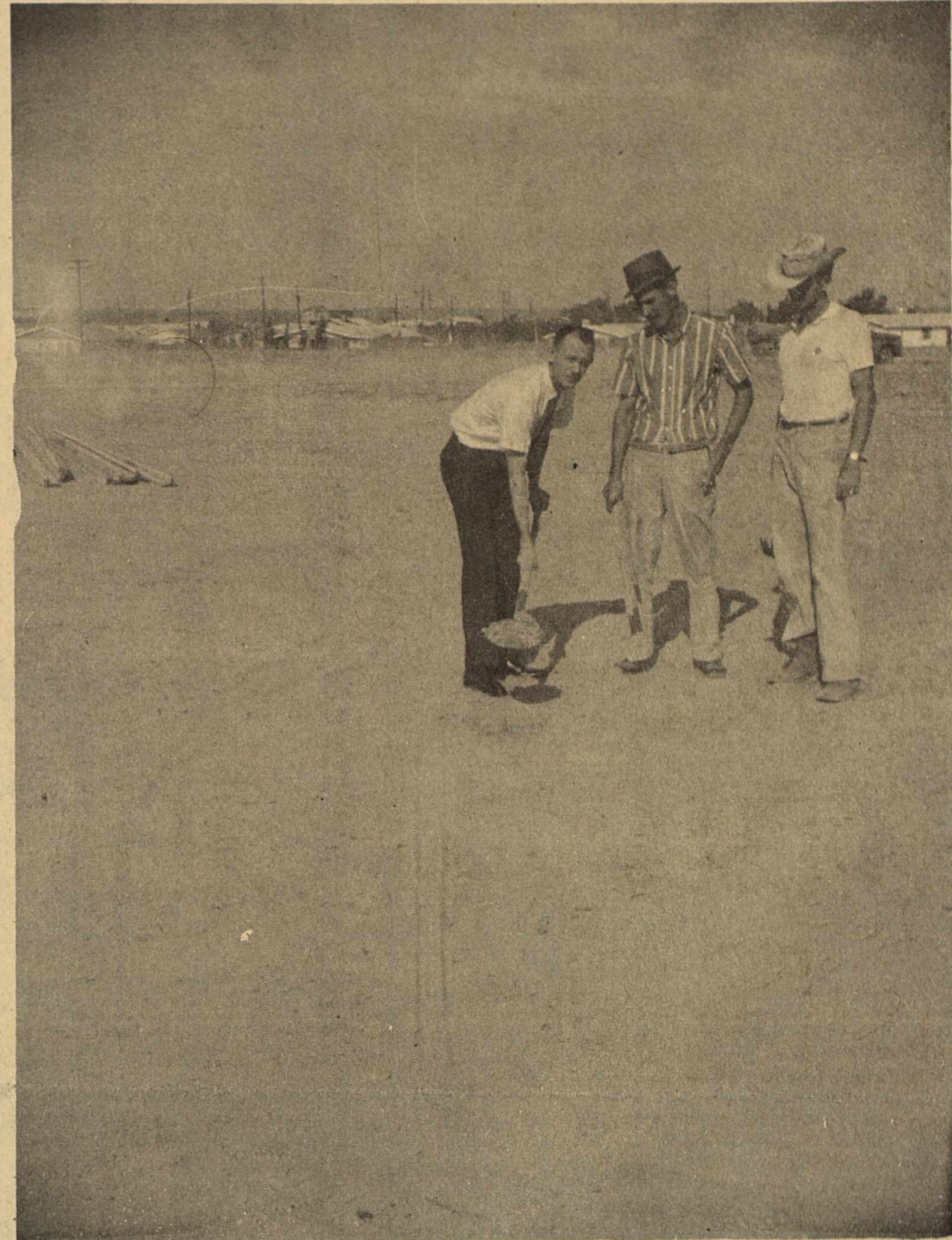
MR. JOHNNIE BROWN---Mayor of Plains and President of the Plains Lions Club spades out the first shovel-full of dirt in several shovel-fulls to follow in what will be the foundation and footings for the new Lions Den-Scout Hut which has just been begun, and on which construction is expected to be completed in about six or seven weeks.
