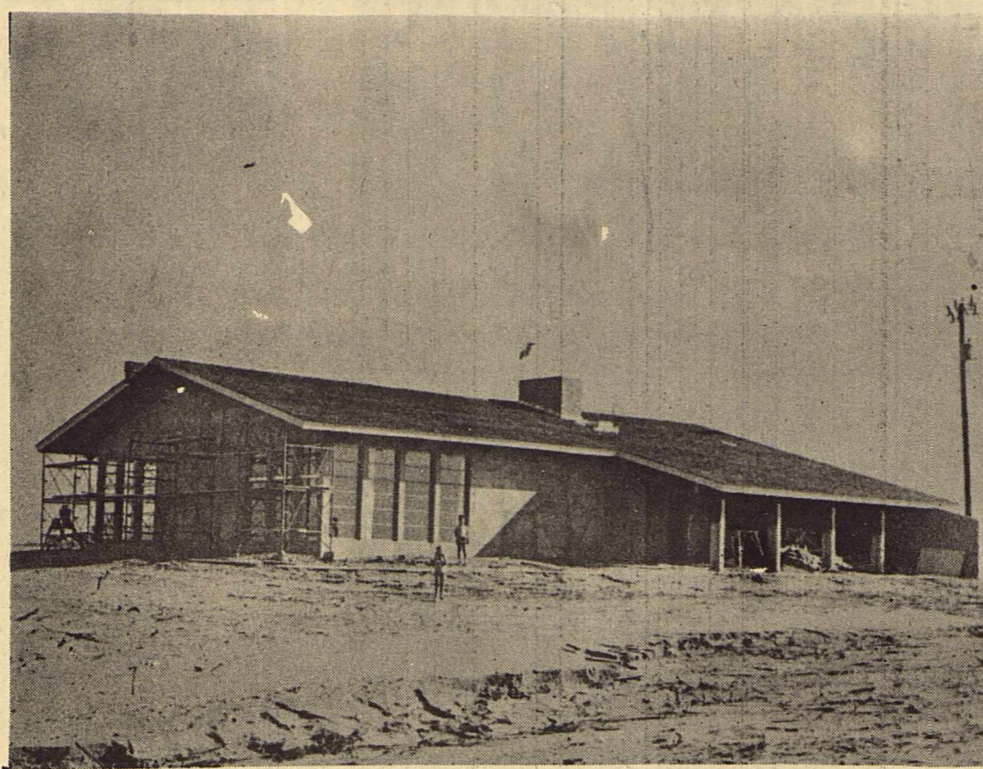
THE CLUB HOUSE AT THE COUNTY PARK NEARS COMPLETION
