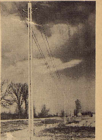
SLIM & TRIM... Installed in a Detroit suburb, these "see through" wood utility poles are among new designs that will appear as the pole industry and electric utility companies make their contribution to national outdoor beautification.
