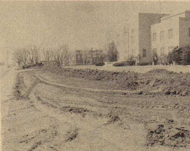
PARKING AREA STARTED
