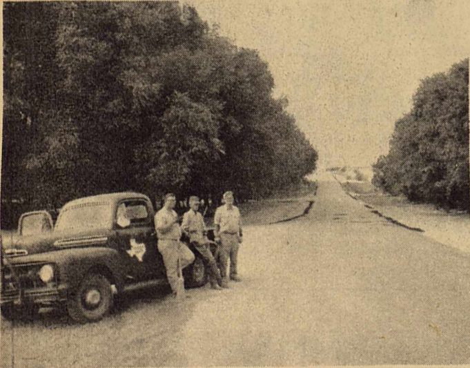
Street repairs made before repotting.
