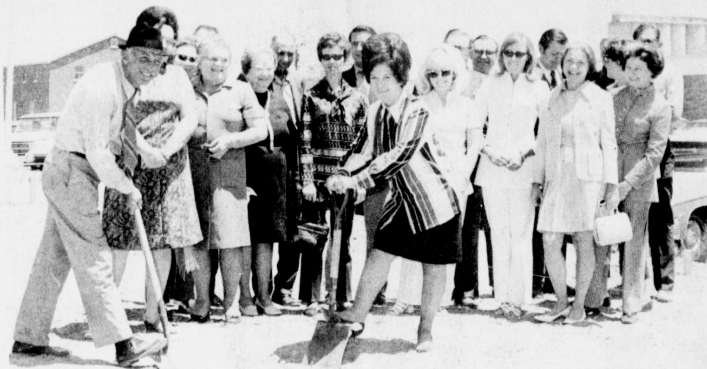
MAYOR AND LIBRARIAN AT GROUNDBREAKING--Officially performing the ground breaking for construction of a new building to house the Muleshoe Area Public Library were at left, Irvin St. Clair, mayor of Muleshoe and Ann Camp, librarian at the Muleshoe Area Public Library. Shown watching are several members of the city and county officials, civic clubs, Friends of the Library and Library Board members, Bill Cantrell, architect from Lubbock, and Jerry Gailey, contractor also of Lubbock. Work is now officially underway on the building site at West Second Street and West Avenue D.
