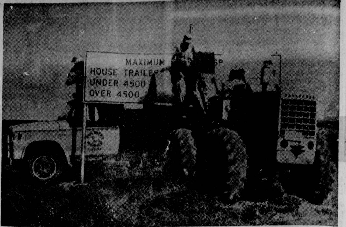
IT'S NOW OFFICIAL — Speed limits were boosted to 70 mph in Bailey county, and throughout much of Texas, Friday, and here several huge gateway signs, listing the new speed limits. This one was being placed on SH 1360 between Arch, N.M. and the Tex-workmen are shown as they put up one of as line. (Journal Photo & Engraving)
